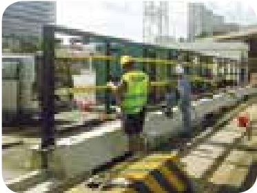
Standardized concrete foundation and steel structure to mount conductor rails
