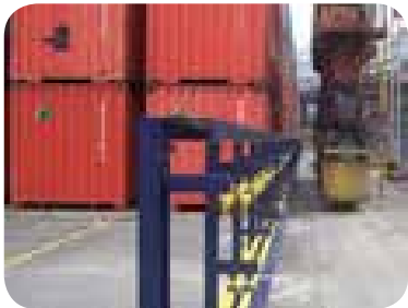
Steel structure and conductor rails for one container block to provide the electrical current – the 2+2 version
